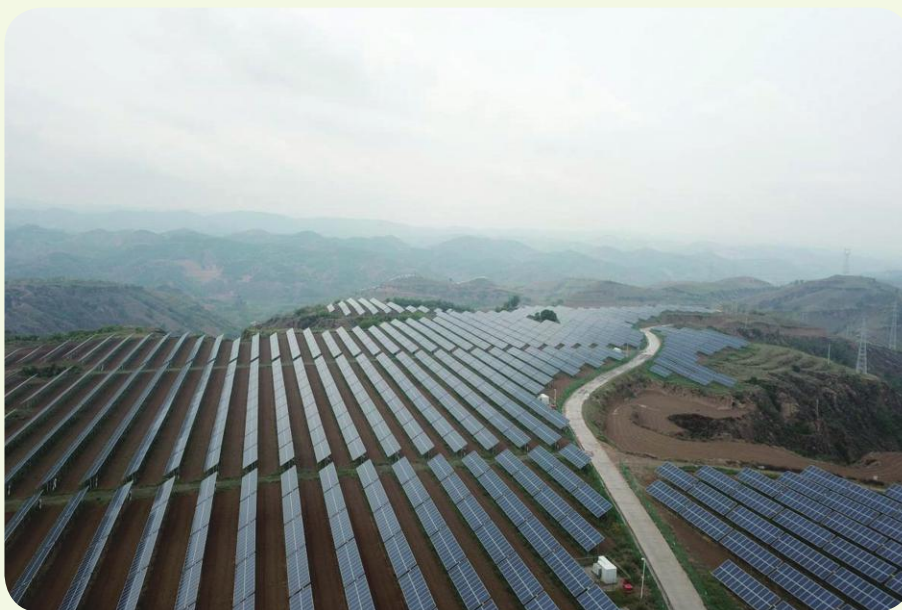
▲ Photovoltaic power station in Shilou County
