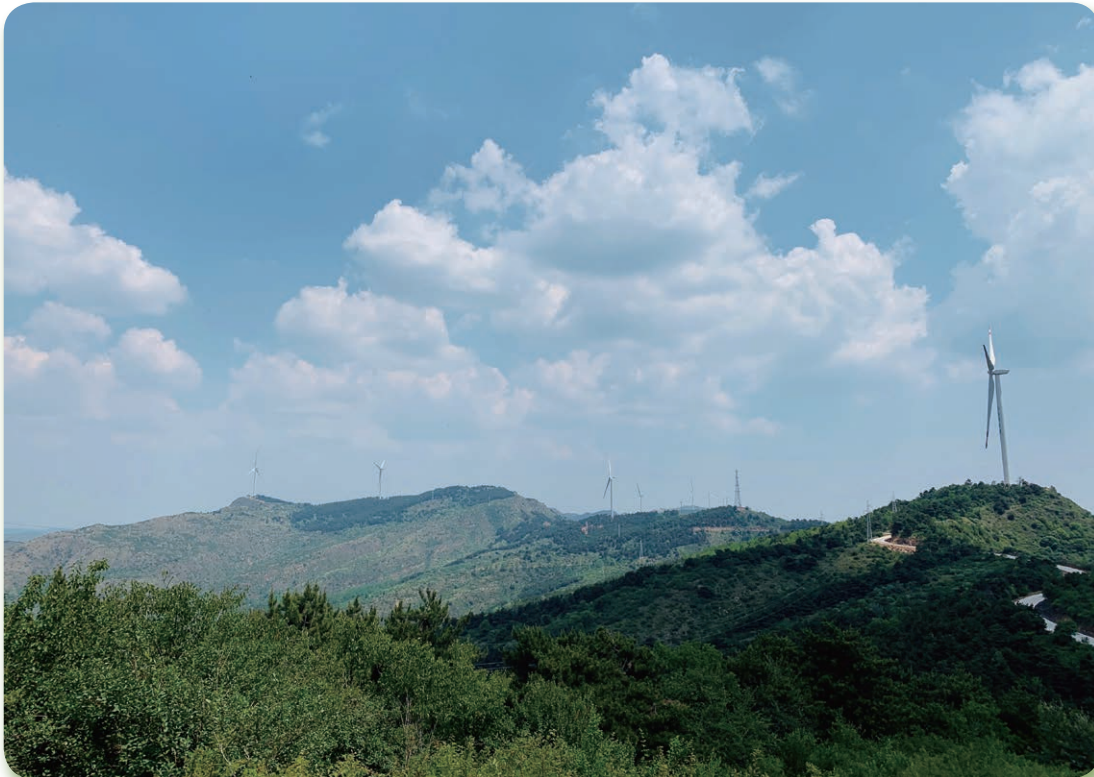
▲ Fengning Wind Farm
